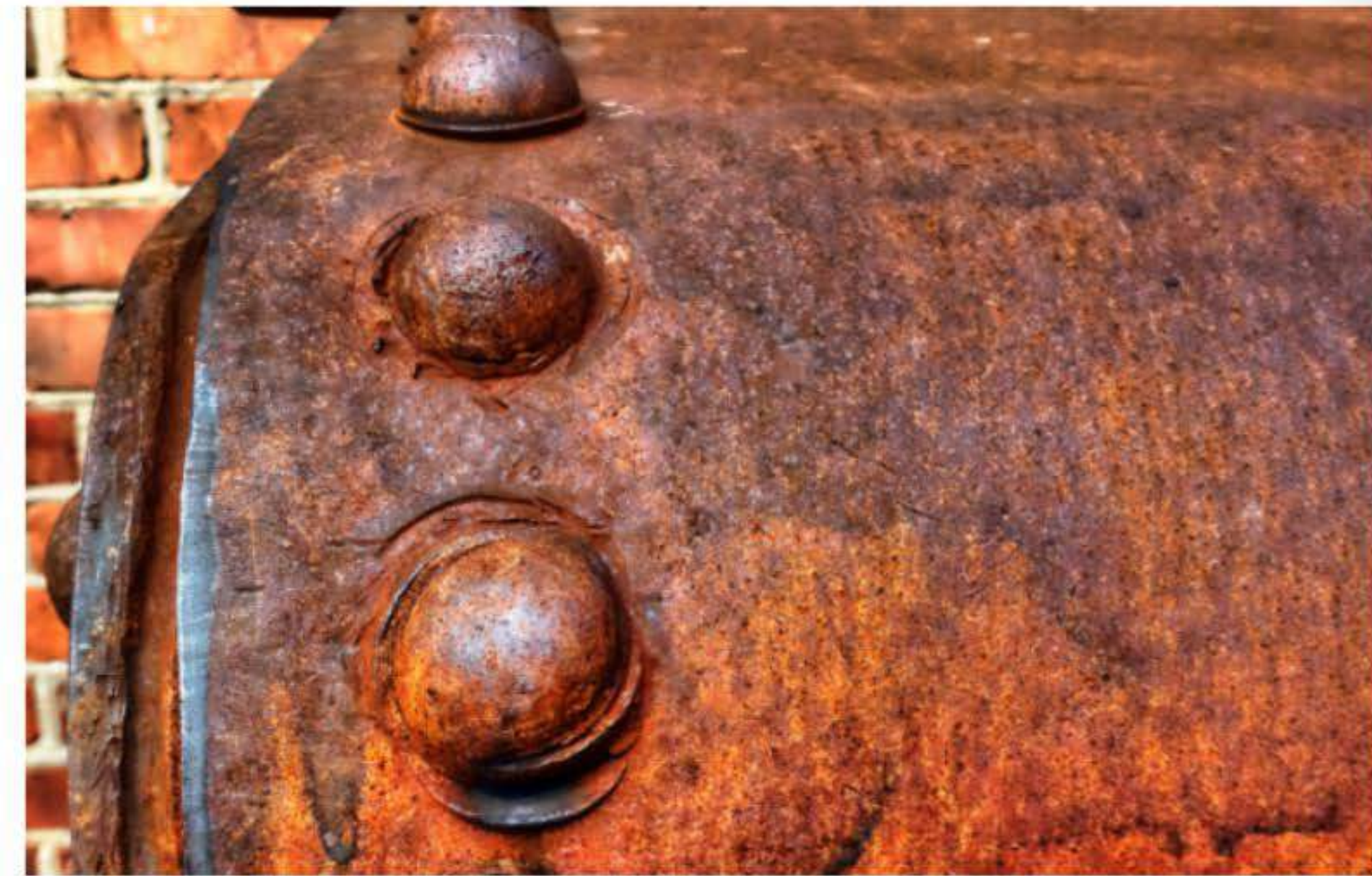
alter Dampfkessel September 2018
